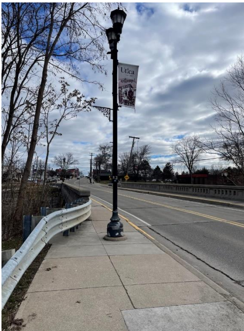
Figure 54: Auburn Road Bridge Over Clinton River Facing E; N Side of Auburn
