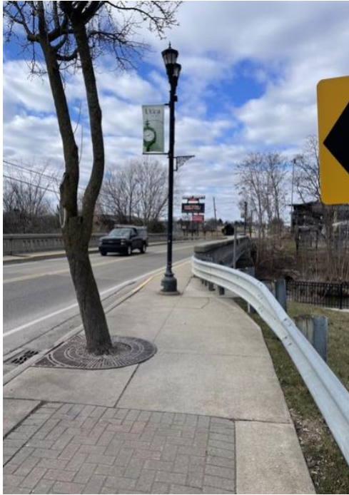
Figure 68: Light Pole Impeding Sidewalk Over Bridge Before
