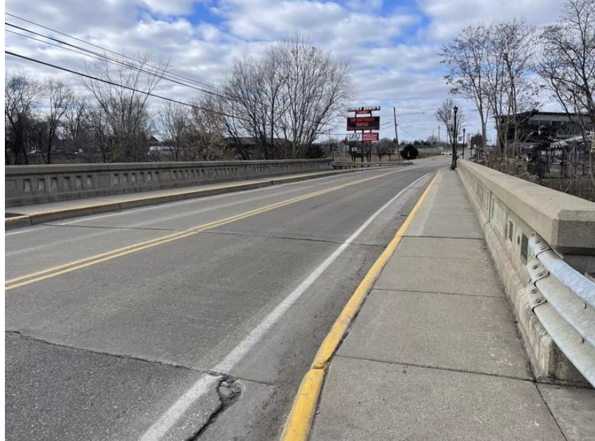
Figure 70: Bridge Over Clinton River Before
