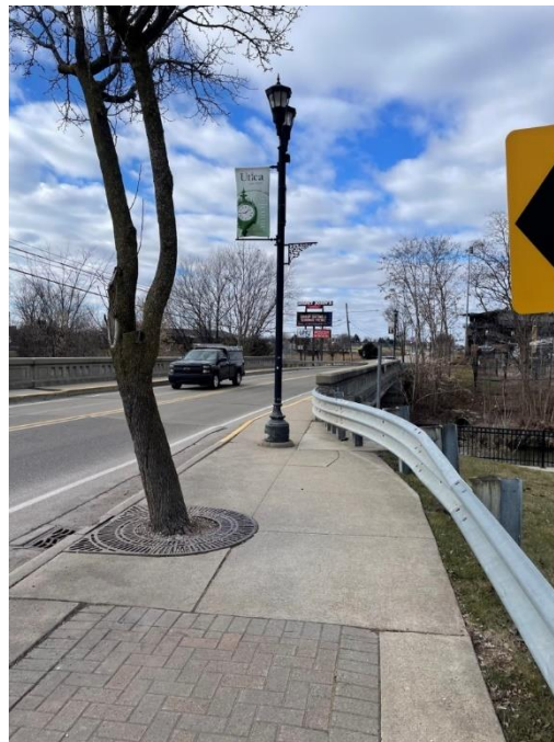
Figure 55: Auburn Road Bridge Over Clinton River Facing W; N Side of Auburn
